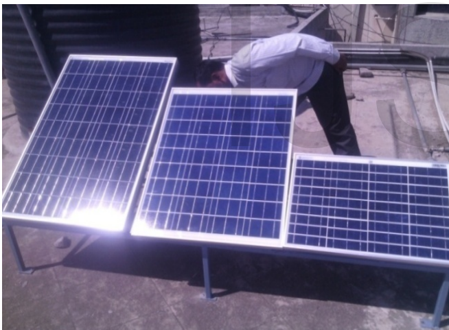
Fig.5 Solar panel installation on the terrace
